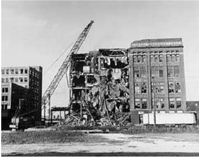
Wrecking a Swift Company building in the Union Stock Yards.
